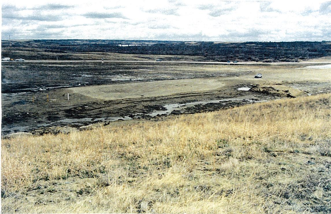
Fig. 12. Looking north at the open excavation east of the bridge structure showing seepage from the intertill gravel in early May 1997.
