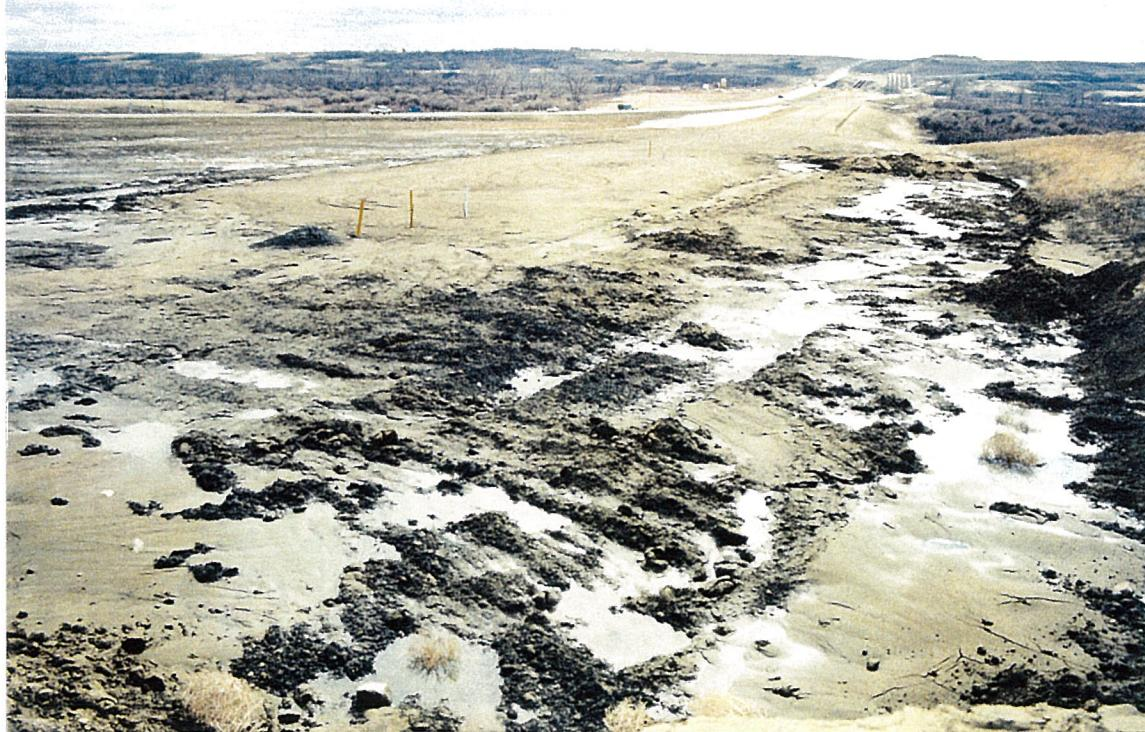
Fig. 14. Seepage in south ditch east of the underpass structure in early May 1997.
