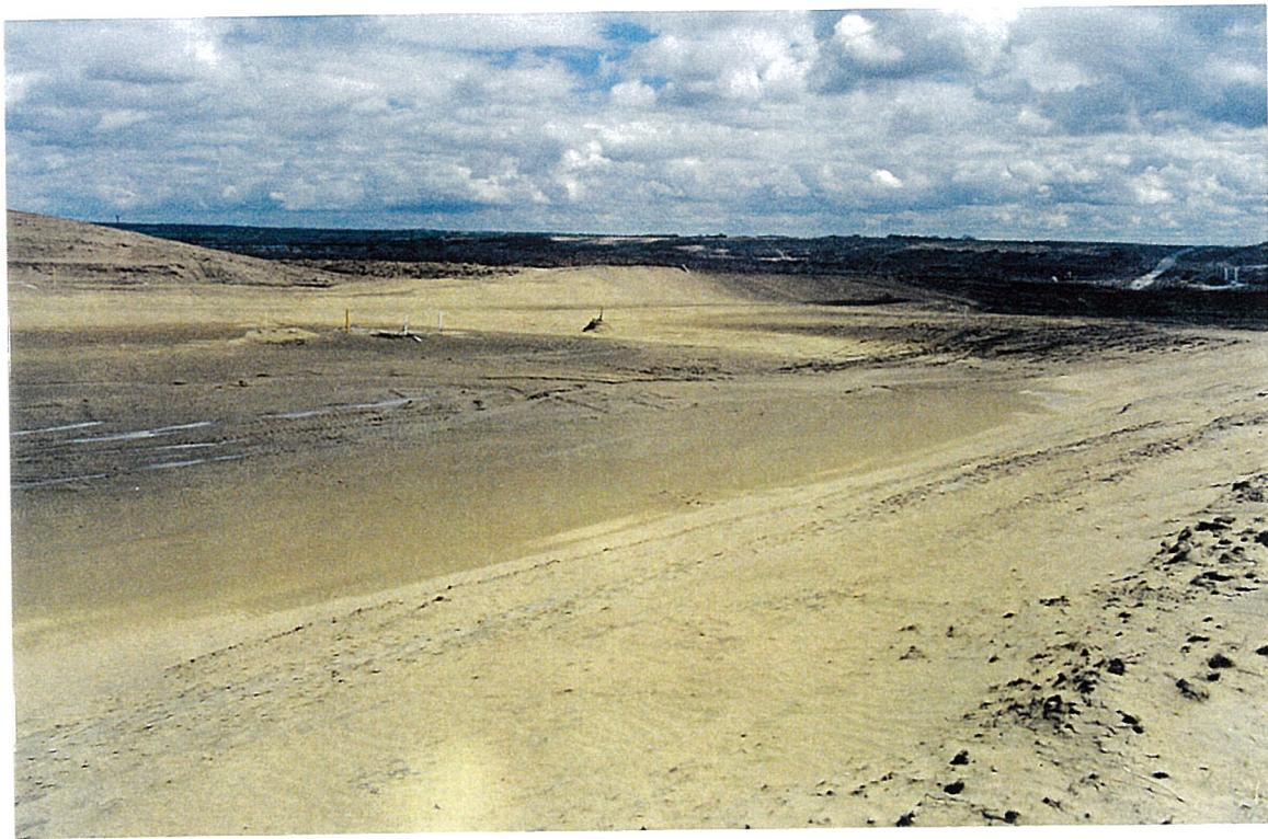
Fig. 21. Unstable ground in wet areas where head in the surficial sand is near the ground surface west of the underpass structure in early May 1997.
