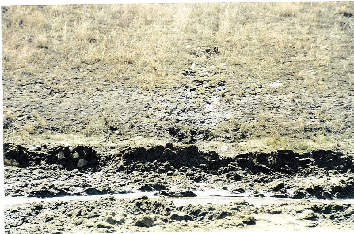
Fig. 15. Seepage from south backslope east of the underpass structure in early May 1997.
