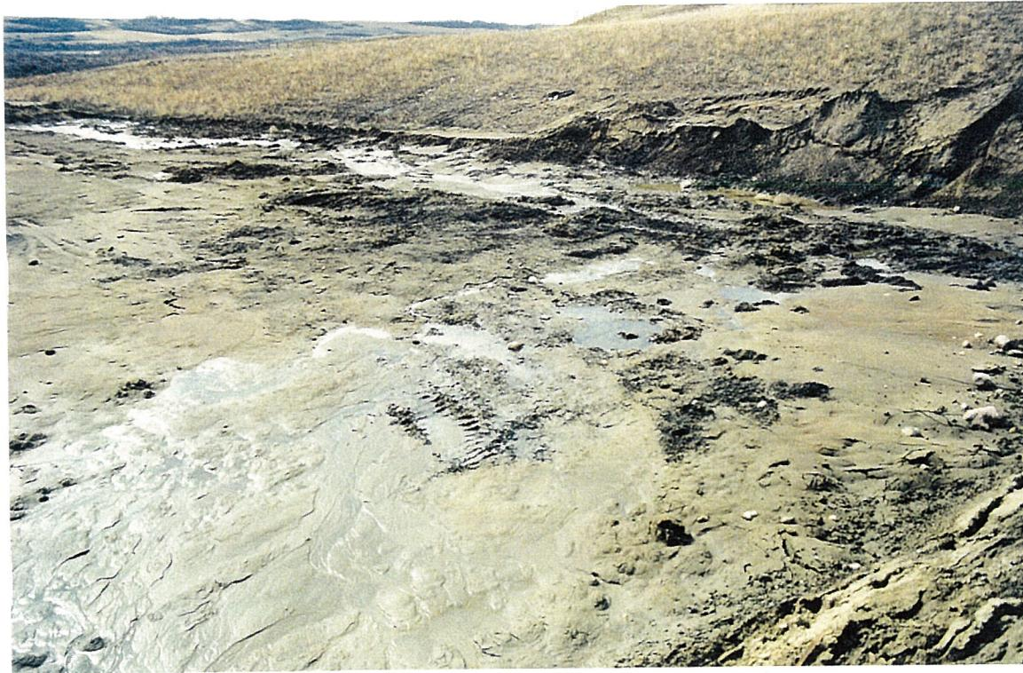
Fig. 13. Seepage in south ditch east of the underpass structure in early May 1997.
