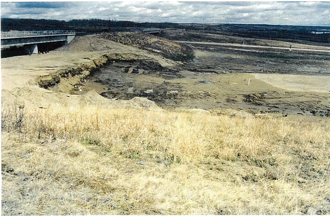
Fig. 11. Looking north at the open excavation below the bridge structure showing seepage from the intertill gravel in early May 1997.
