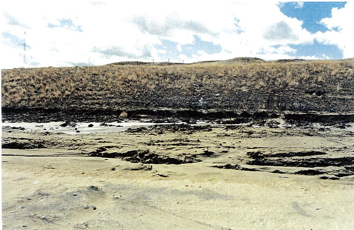
Fig. 16. Erosion from Seepage from south backslope east of the underpass structure in early May 1997. Seepage apparently from intertill gravel above Dundurn Formation.
