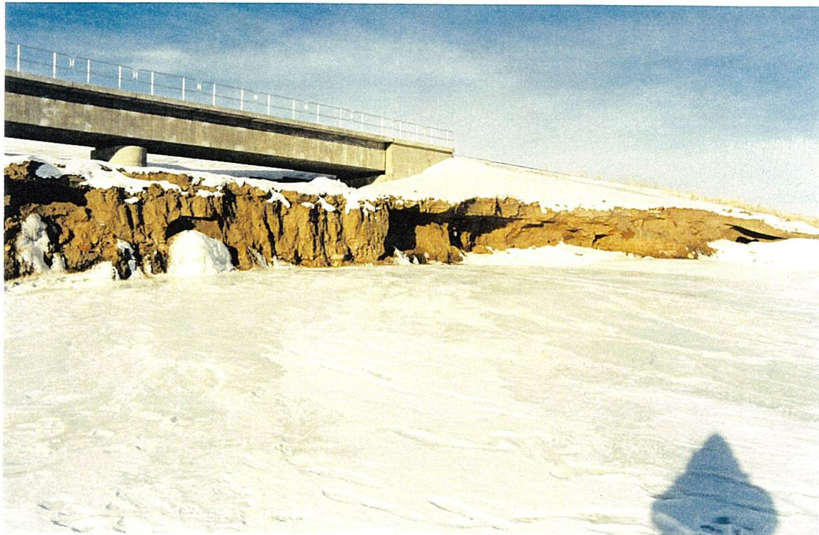
Fig. 8. Looking west from the underpass in February 1997. Ice buildup from groundwater seeping from the intertill gravel and surficial sand.
